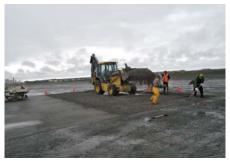
Raking out and compacting the base material to provide a solid, well drained foundation for the Endura-Form installation
