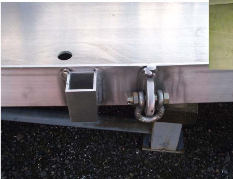
**Figure 02:** A closer view of the railing post socket, the lifting lug and shackle and one of the drain holes. The side is 4" high. There are four lifting lugs and shackles are 2.5 ton capacity and has a cotter pinned nut and bolt. Total weight of the completed 20' walkway is less than 1000 lbs.
