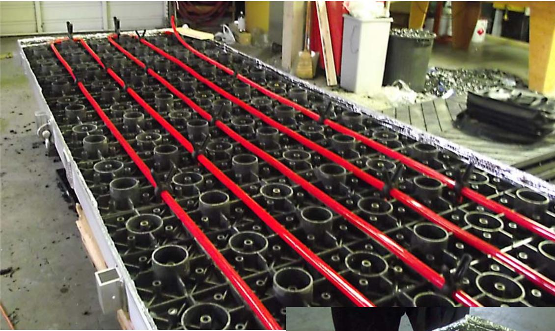
**Figure 07:** This image shows the heating lines laid in place at 8" intervals. Five lines are fitted, the sixth is not yet in place.
