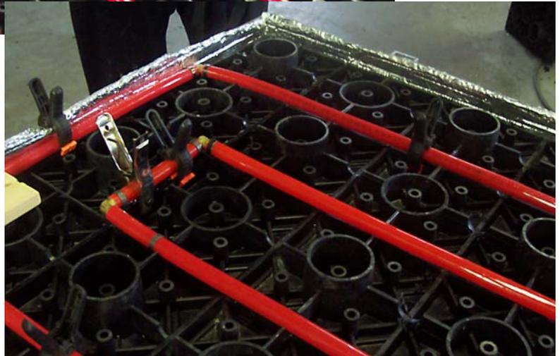
**Figure 08:** A closer look at the crimped brass fittings that connect the various lengths of heating line. The crimping rings are specially designed to work with the Oxyplex heating lines.
