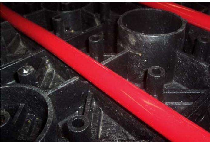
**Figure 06:** This close up shows how the 3/4" Oxypex heating lines travel through channels in the Endura-Form panels. The lines will be securely sandwiched in place when the top panels are put in place.
