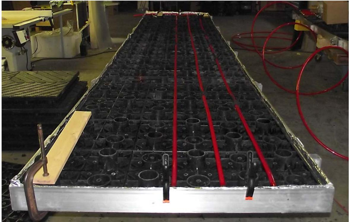
**Figure 05:** The bottom layer of Endura-Form panels are laid in the tray and the task of fitting the heating lines starts. The lower layer of panels are fitted with fixed receiving nuts for secure fastening of the top panel layer. The bottom panels are also fitted with drain holes (100 per panel) to allow proper drainage of the interior of the panel assembly.
